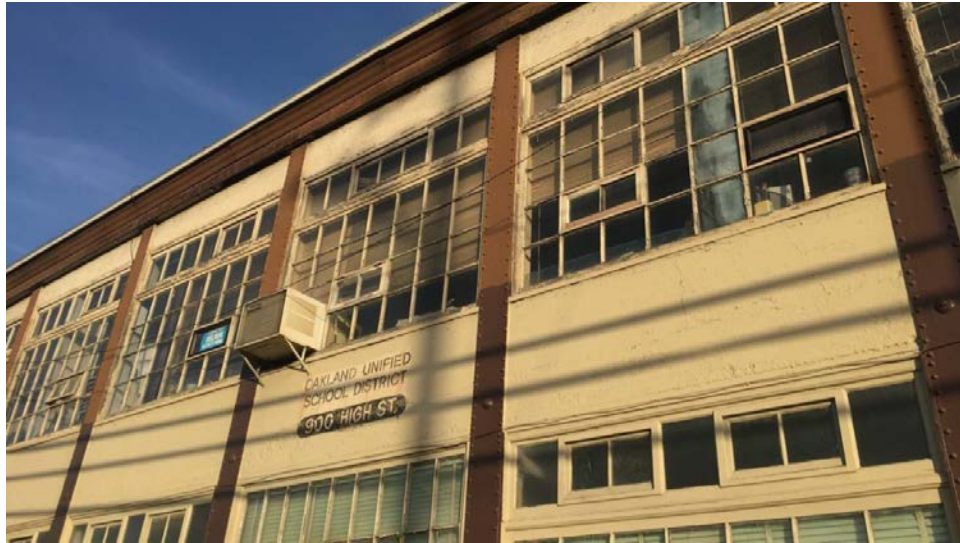
Figure 17: OUSD administrative building
